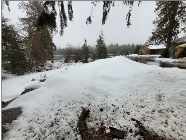
Photo 3. Fill placement along west side of Laird Creek and proposed alignment of lower fencing area.
