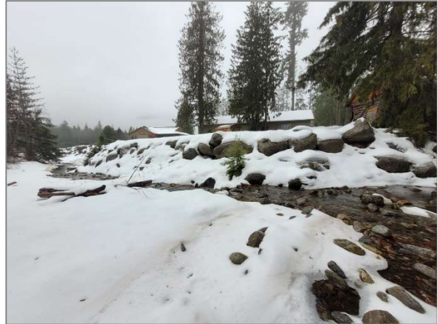
Photo 4. Angular rock placed along west bank of Laird Creek below placed fill.
