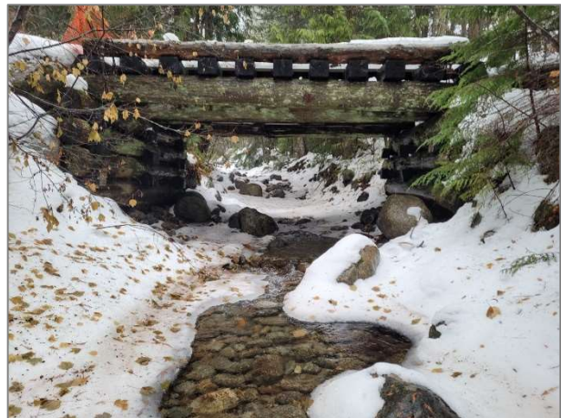
Photo 6. Upstream view of old timber bridge crossing Laird Creek.
