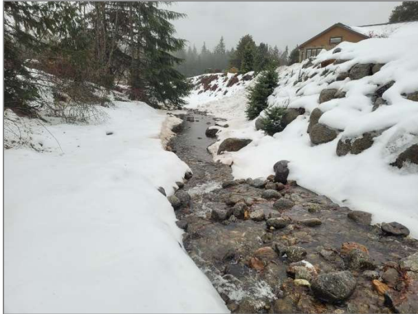
Photo 9. Downstream view of Laird Creek by lower fencing location, with riprap along bank.
